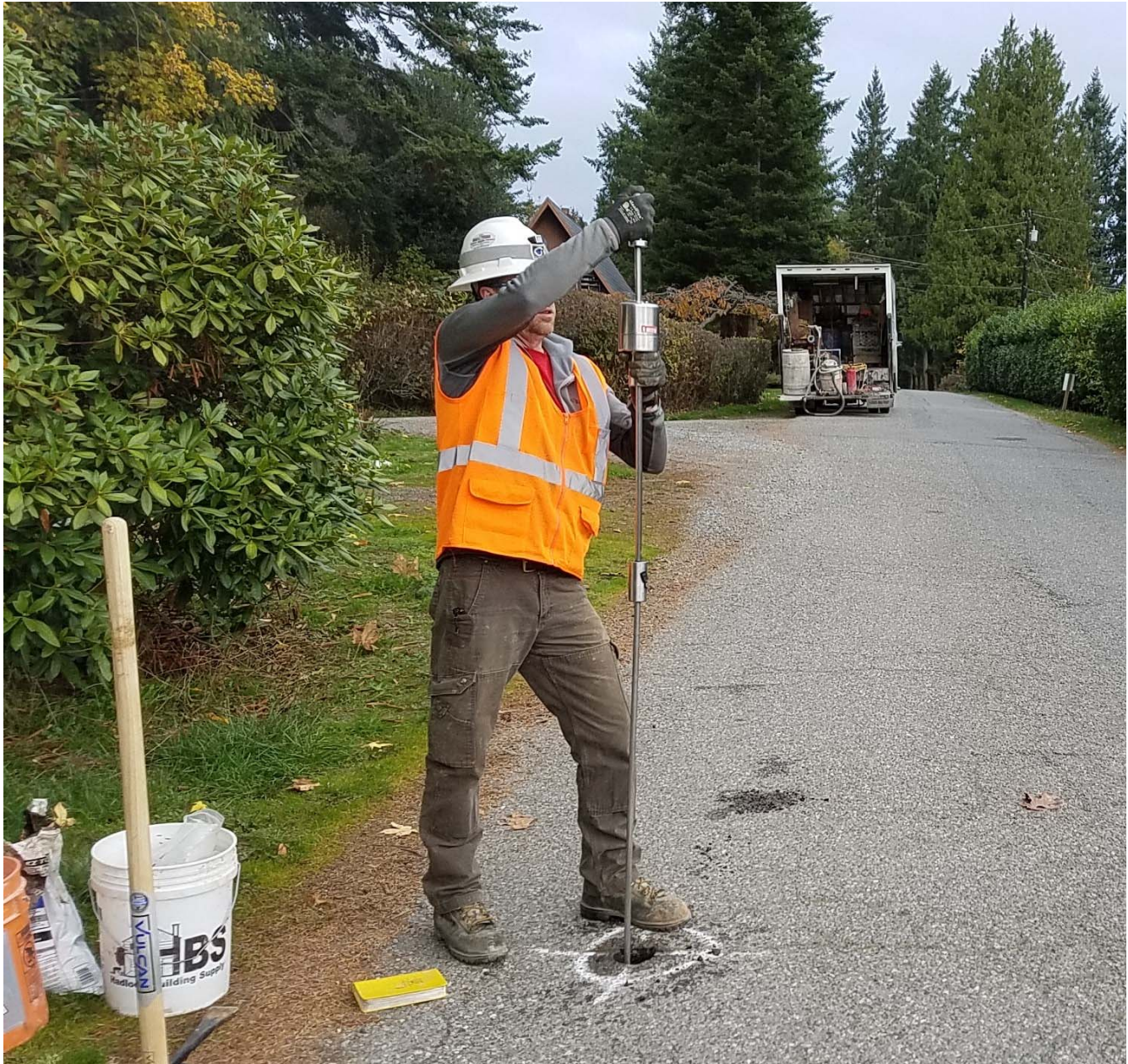
Photo I: MTC Geologist during Kessler DCP advancement at C-12 on 42 nd Street. Facing north.
