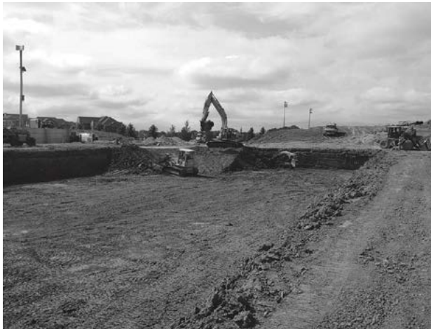
Excavate bed and prepare subgrade per engineer’s plans.
